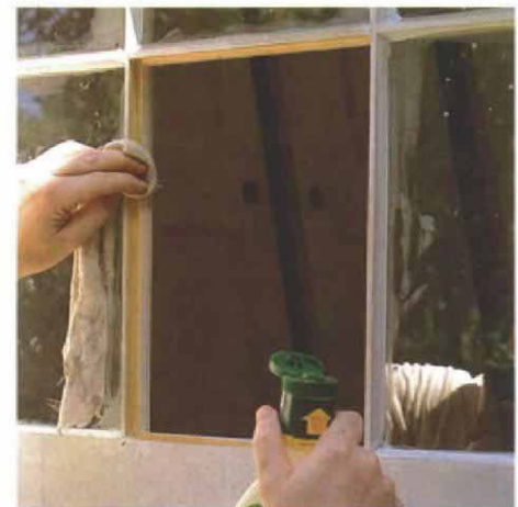
Prep the bare wood with linseed oil. Linseed oil refreshes the wood and keeps the wood from drawing the oil out of the putty.
