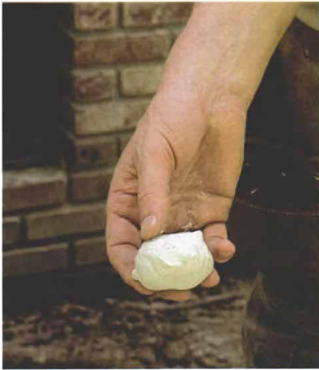
Warming up the putty. Knead a ball of putty about the size of an egg to warm it and make it soft and workable.
